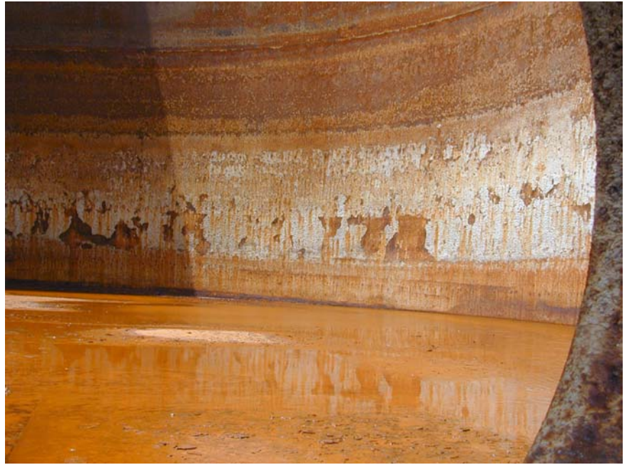
Figure 5. Inner wall of a storm water storage tank.
