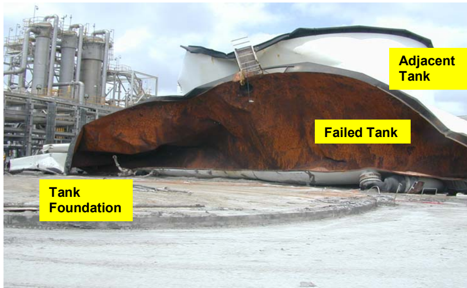
Figure 1. Sides of failed tank lying against adjacent tank.
